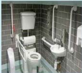
Illustrations 10, 11, 12: Accessible toilet design (BS8300 - 2001); Accessible toilet; Ambulant toilet
